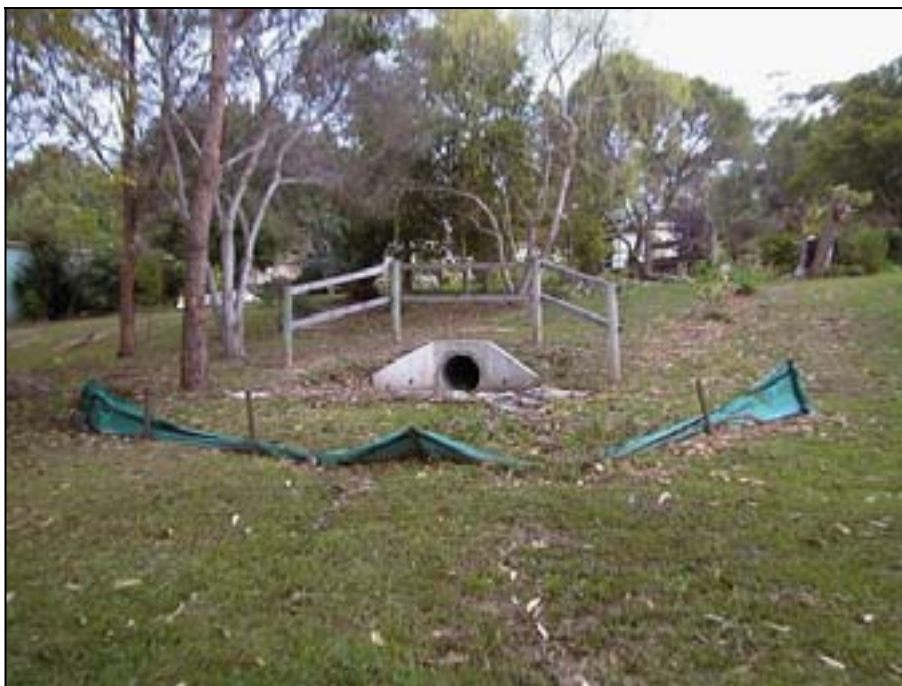
Photograph 1 - Drainage outlet - No. 57 O'Connells Point Rd, Beauty Point
