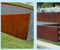
Corten steel blade retaining wall examples
