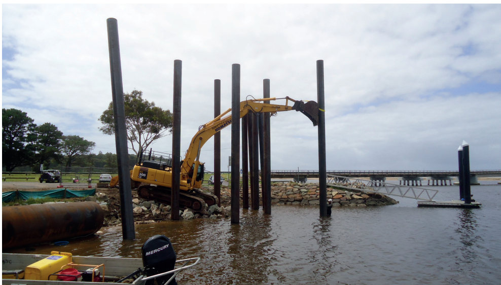
Steel piles being positioned prior to being driven into the river bed to provide footings for the new boat ramp.
