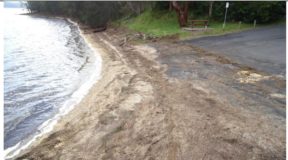
Boat ramp – bitumen above MHWM, then in-situ sand / shell grit below
