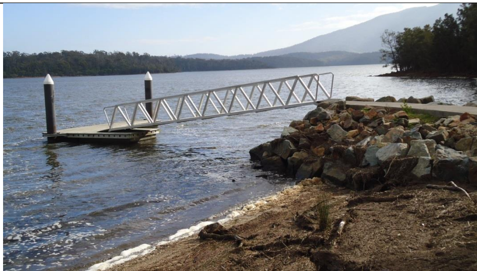
Bellingham pontoon, truss gangway and abutment
