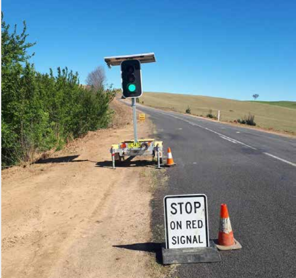
A solar-powered traffic light in use on Mogilla Road.
