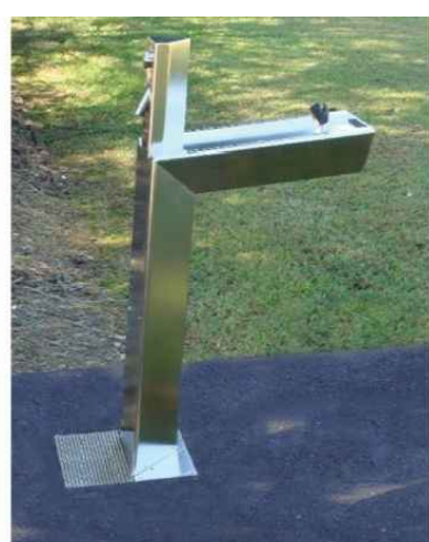
BUBBLER W/ BOTTLE FILL BRAND: AQUAFIL STYLE: BOLD STAINLESS STEEL REFILL STATION QUANTITY: 1 SUPPLIER: AQUAFIL.COM.AU INSTALL: REFER TO MANUFACTURERS INSTRUCTIONS AND SPECIFICATION. CONNECT DRAIN TO SOAKAGE PIT
