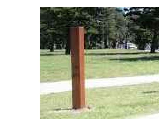
TIMBER BOLLARD HEIGHT: 1000MM SIZE: 200 X 200MM HARDWOOD REFER TO SPECIFICATION
