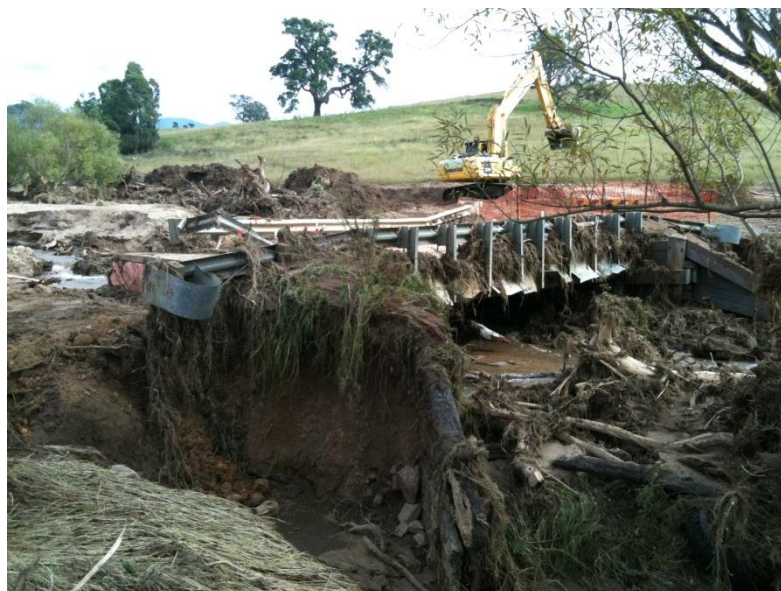
Figure 15.7: Debris and Blockages at Bridges (from Council's Flood Data Library)
